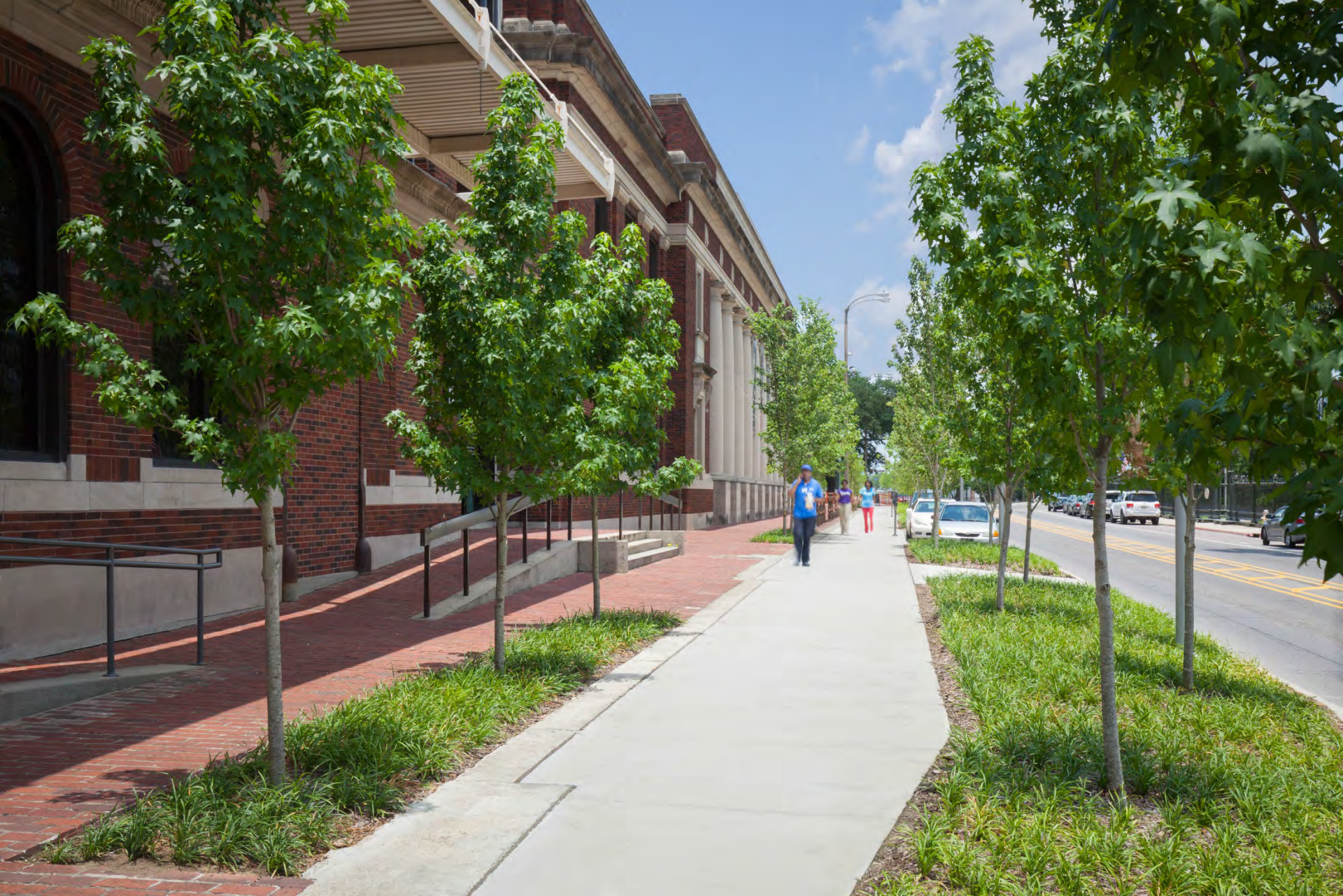
Roadway reduced by 20' and replaced with Multi-use path and native trees
